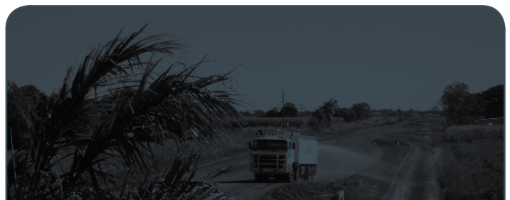
Construction works on the Bundaberg Ring Road
